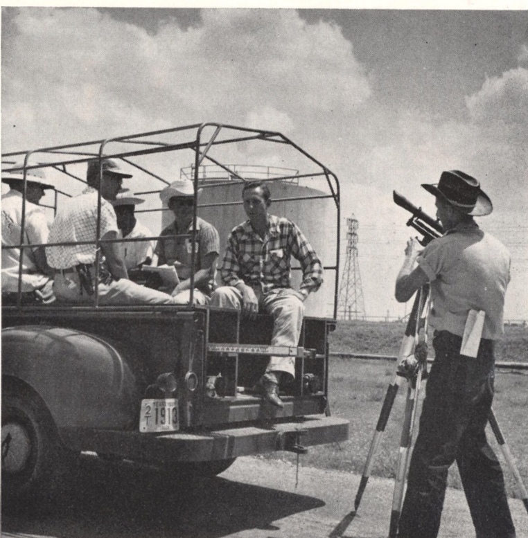
A familiar sight around the Refinery, the red pick-up transports the surveyors from one important project to another.
