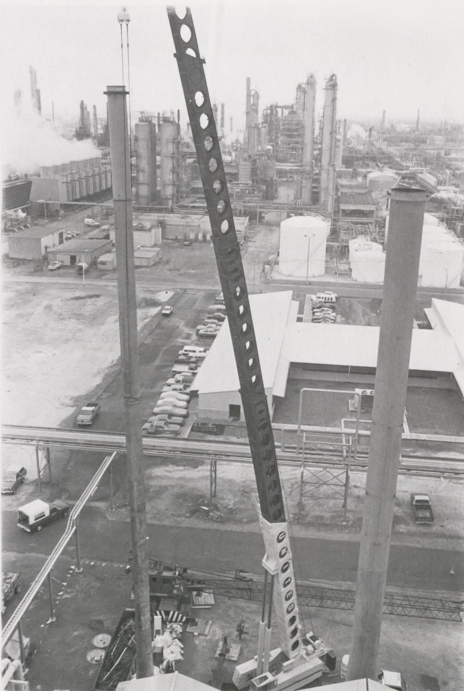
SKY'S THE LIMIT...A 150-foot furnace stack is removed by a crane as part of the MVI debottlenecking project.
