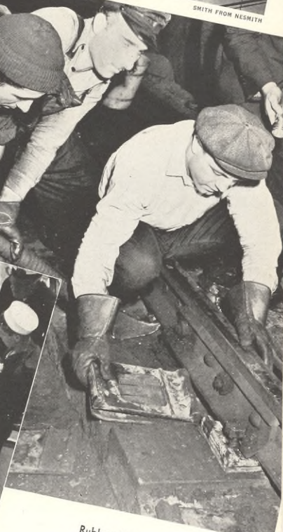
Rubber "silencers" under the rails of New York's subway mean quieter rides
