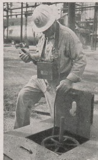
S. A. Martin takes the usual safety precaution of testing for gas in operating area. Work will not begin until he has given "all clear."
