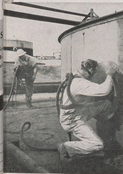
C. Lawrence operates the blower pump as C. Zimmerman begins his inside inspection of a tank. Gas mask guards against fumes.
