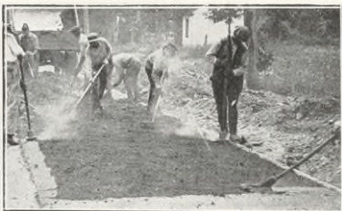
Laying, spreading, and tamping Texaco Sheet Asphalt wearing surface on New Jersey section of Lincoln Highway.
