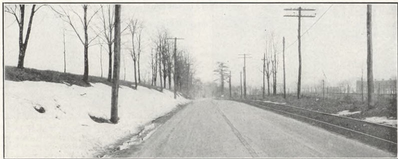
Completed Texaco Sheet Asphalt on a section of the Lincoln Highway
