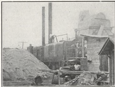
Railroad type of asphalt plant on New Jersey Lincoln Highway paving job
