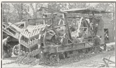
Rotary excavator ripping up surface of old road preparatory to grading and resurfacing
