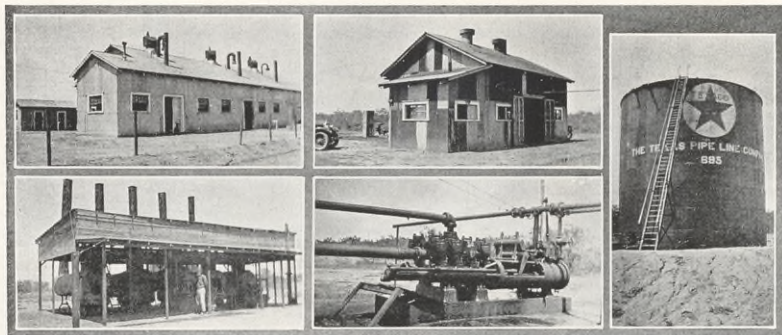
Above: 1. Wilson Ranch Pump Station, Holliday District 25. This Station has three units: two 100 h. p. Primms and one 80 h. p. Primm engine. The small house at the rear is the air compressor house. 2. Nichols Station, Holliday District 25. This is a one unit station.
