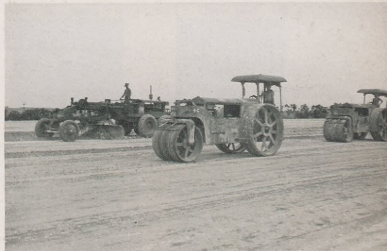
Men of an aviation engineer battalion pack coral with pneumatic rollers to make a base course for asphalt.
