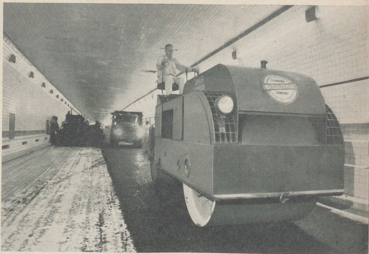
One of the two rollers used by the Standard Bitulithic Company in paving the new Lincoln Tunnel tube packs down the first of two layers of asphalt.
