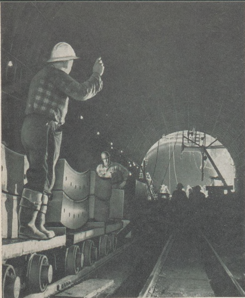
These electric rail cars were used to haul construction materials through an air lock to the tube working area.
