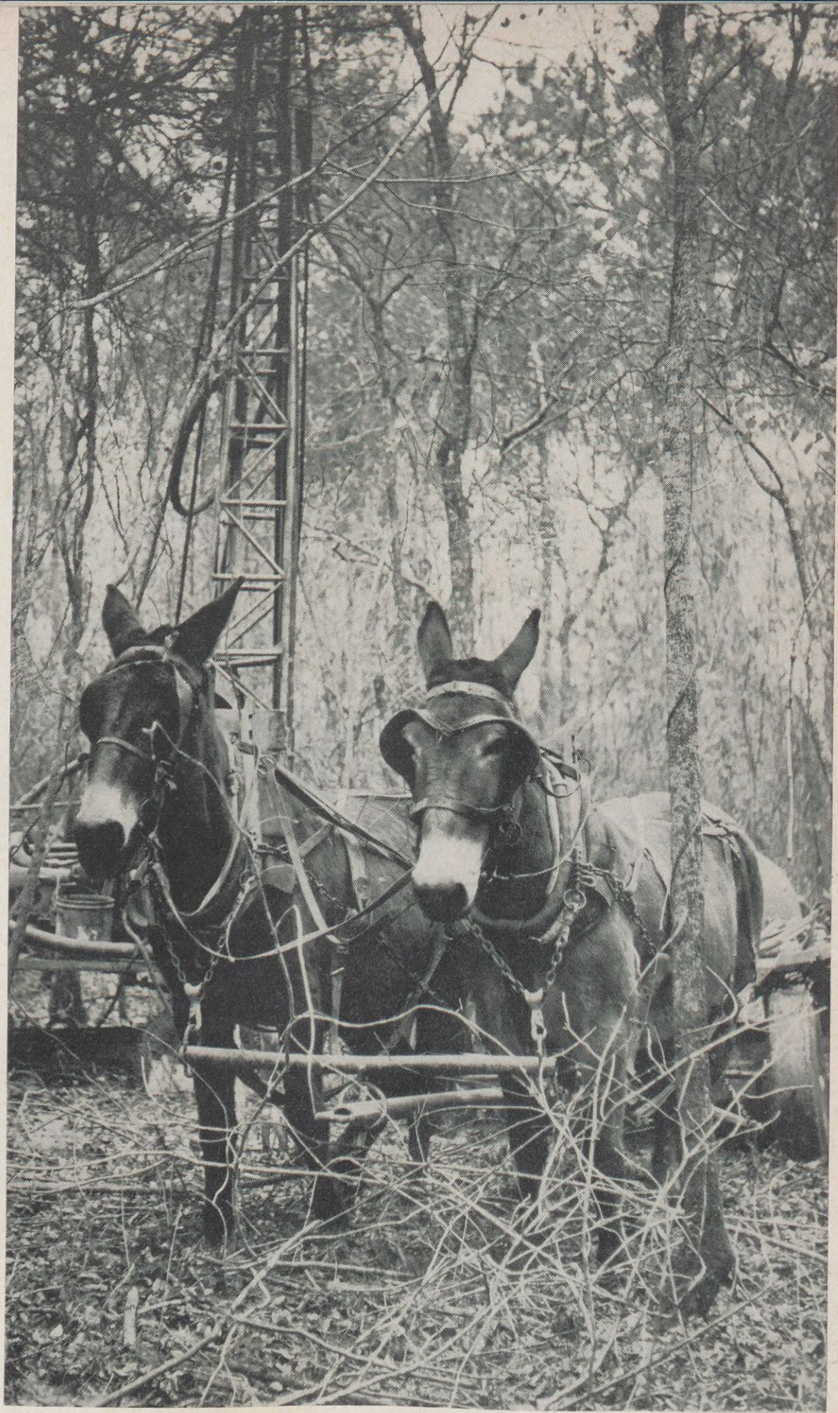
The mule team hauls the wagon carrying the portable drill through heavy woods toward the next shot point. The wagon is equipped with a motor to power the drill.
