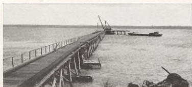
Completing T. T. Co. Wharf at Matanzas, Cuba
