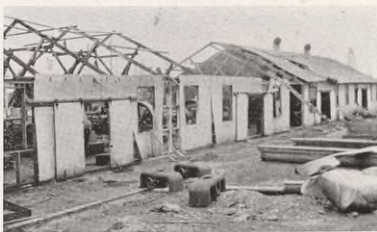
Result of explosion of gas Plant of Chas. F. Noble Refining Co. in N. W. Burkburnett Field.
