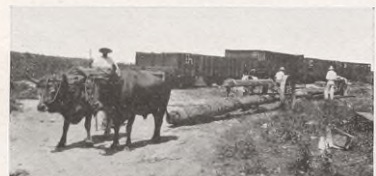
Hauling 80-ft. hardwood piles for our Matanzas Wharf
