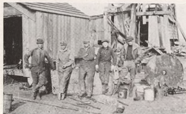
Rigging-up Crew on Myers Well
