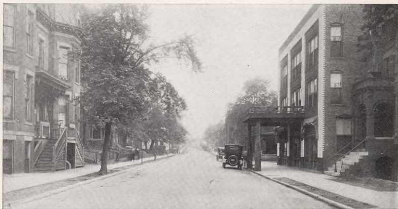
Cherry Street, Kansas City, Mo.—Old brick pavement surfaced with Texaco Asphalt in 1911—Photograph taken in 1919
