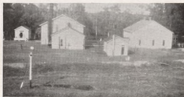
Dayton, Texas Pipe Line Station
