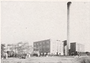
Texas Power and Light Company, Waco, Texas Waco Generating Station
