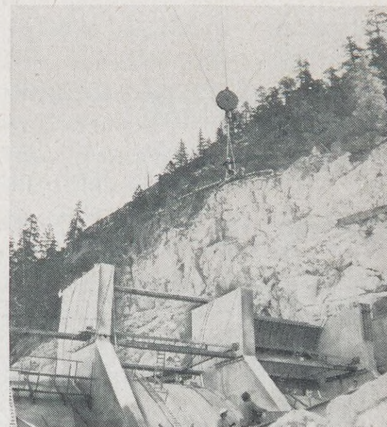
Giant hoist delivers materials to gate-controlled overflow spillway at Donnell's Dam.
