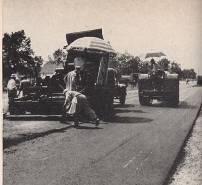
ON THE HIGHWAY, workmen lay a thick surface of heavy-duty Texaco Asphaltic Concrete, one of the most durable pavements today
