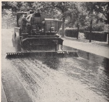
IN THE CITY, this pressure distributor sprays on a surface treatment of Texaco Cutback Asphalt to form a waterproof, dustless mat
