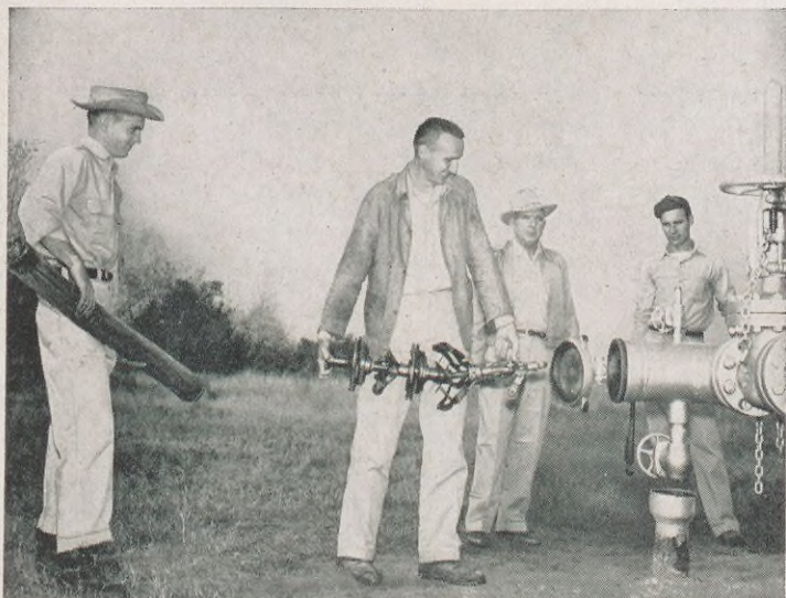
Leadman J. H. Starks prepares to insert a scraper-type pipe line cleaner into a products line as Pipeliner J. D. Andersen stands by with a log to push it in. Looking on are Maintenance Foreman C. C. Moss (wearing hat) and Pipeliner J. S. Broomas.
