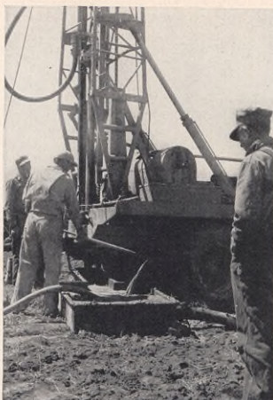
DRILLING A SEISMIC SHOT-HOLE
