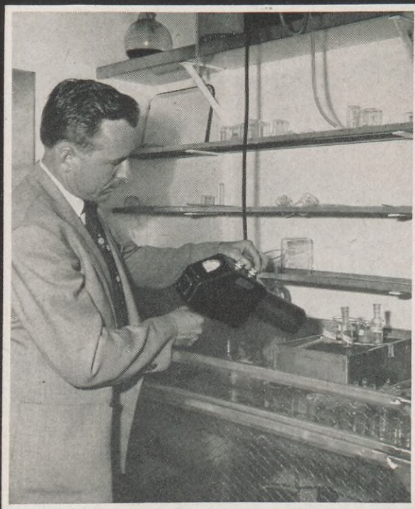
Amount of radiation coming from contaminated laboratory glassware is measured by Safety Inspector R. J. Shreve, of Emeryville's Safety and Industrial Hygiene section, with an ionization chamber.
