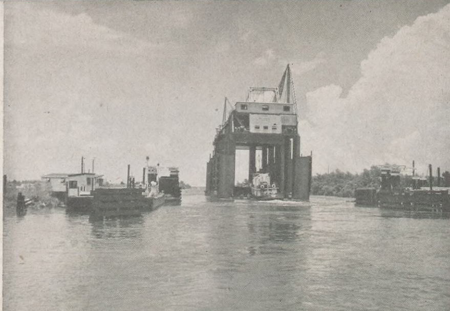
Down to the sea on stilts. With one tug pushing in the drilling slot and another pulling, the ODECO rig heads for a Shell lease in South Pass, Block 27, to drill its first well. The derrick is folded down while the barge-mounted platform is afloat.
