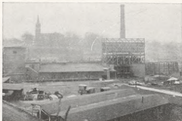
Carolina Public Utilities Corporation—Columbia, S. C. plant
