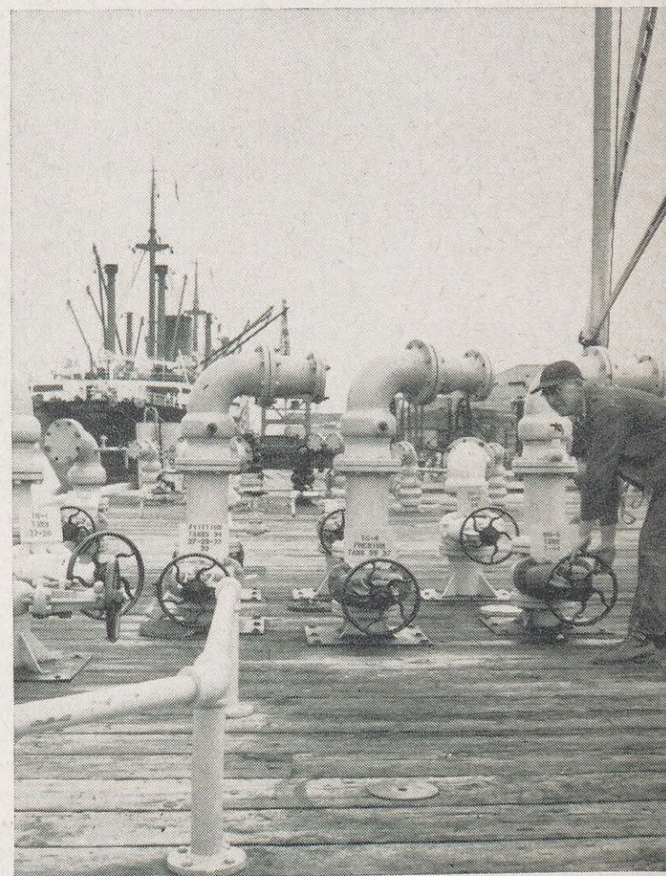
H. J. Williamson, Gauger-Dockman, adjusts a valve on the tanker berth at the Harbor Island Terminal. Lines from tankers are connected here and products are pumped through the valves to storage tanks ashore.
