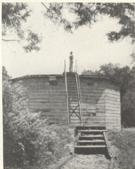
Chief Clerk M. B. Burks on a storage tank in the field. Tanks of wood are enclosed to prevent the sun's opening seams
