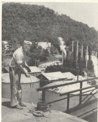
Gauger Arthur Metcalf gauges a storage tank. Much of the refinery is on a hillside, providing some gravity flow of stored crude
