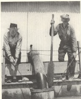
Machinists Second Class W. F. Smith and R. L. Kelley clean strainers on pipe line through which water is pumped from river to refinery
