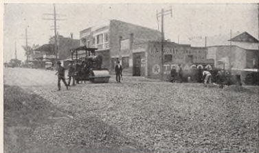
Texaco Asphalt in Australia Being laid on Lane Cove Road, Municipality of Willoughby, Chatswood, one of the main arteries of Sydney, Australia. The penetration method is being used.
