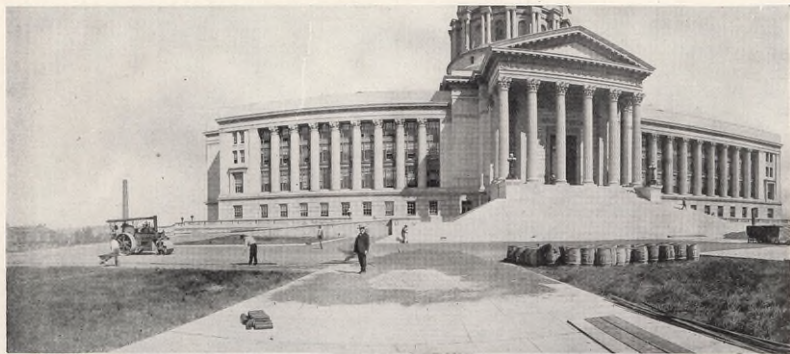
Jefferson City, Missouri Constructing Texaco Asphalt macadam in front of the State Capitol at Jefferson City.
