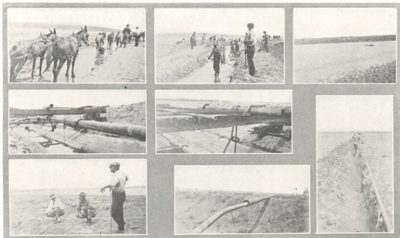
Pipe Line construction work in bed of Red River southeast of Burkburnett in District 14. Taking up 8" line and relaying it on account of the current. Photographs by F. S. Reid.
