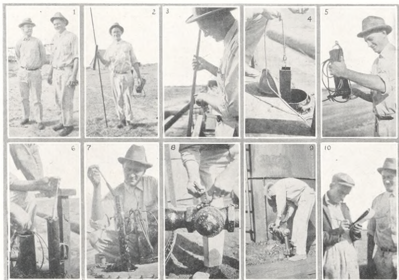
1. Gauger J. B. D. Woodburn and Assistant Gauger R. E. Paullus, Holliday District 25, Holliday, Texas. 2. A gauger's equipment—gauge pole, oil thief, hydrometer, and hydrometer testing case. 3. Reading the gauge pole. 4. Lowering thief into tank to take sample to determine percent of BS and water in the oil. 5. Reading the percent of BS after thiefing a sample of oil. 6. Reading the hydrometer. 7. Taking readings for temperature and gravity. 8. Sealing lock stop on tank, preparing to run oil into line. 9. Locking and sealing tank when running oil into line. 10. Producer's witness signing gauger's run ticket after oil has been gauged.
