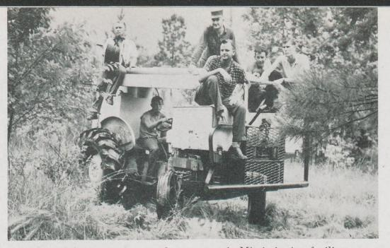
Seismic equipment is mounted on tractors in Mississippi to facilitate travel through densely-wooded areas. Above, members of Shell's Seismic Party No. 31 ride aboard a tractor to a new shot point. They are, left to right, E. K. Crow, D. L. Biles and H. E. Brumfield (all contract "jughustlers"), Shell Party Chief E. P. Cooper (in checked shirt), contract recording foreman C. E. Knippers and Shell Seismologist J. C. McClimans.
