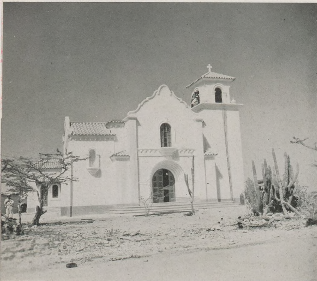
The architecture of Cardon's new church is Spanish in style.
