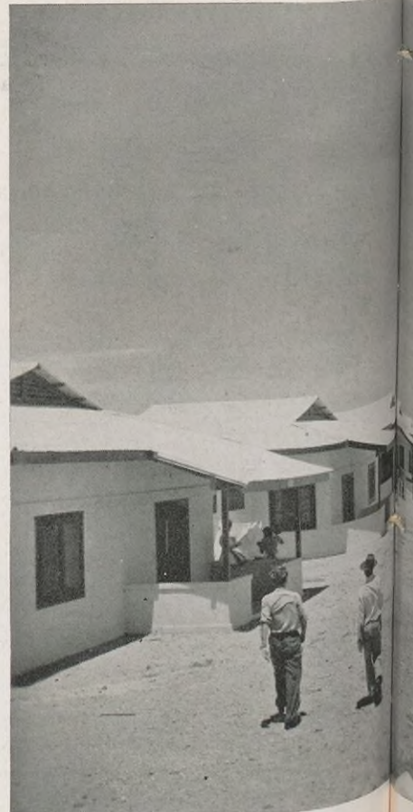
A view of some of the 550 dwelling units
