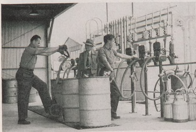
Products from nearby storage tanks are transferred to drums at the new filling rack at San Diego to facilitate distribution. O. J. Graves, Plant Supt. (center), watches Yardmen G. A. Pearson and S. W. Ruhl.
