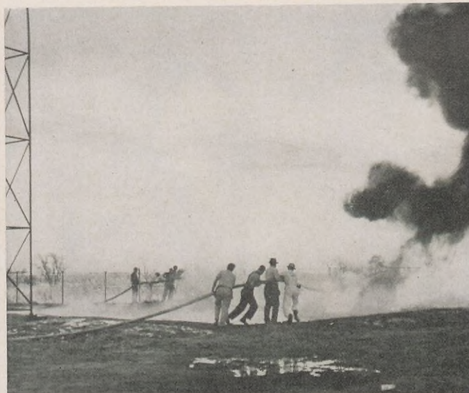
These pictures tell the story of how a 40 x 40-foot pit fire was handled with two fog nozzles. The use of fog (a fine water spray produced by special nozzles) is one of the most effective means of handling a wide variety of oil fires.
