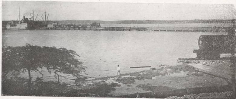
S. S. "Alabama" Discharging at Cienfuegos, Cuba—view from Plant of The Texas Company (So. Am.) Ltd. 1700 feet of 12-inch line connect the tanks with the dock.
