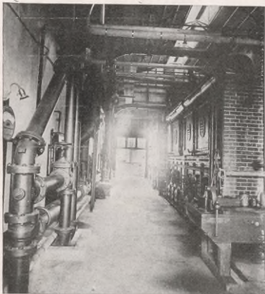
Pumping plant on Pierce Estate, Wharton, Tex.
