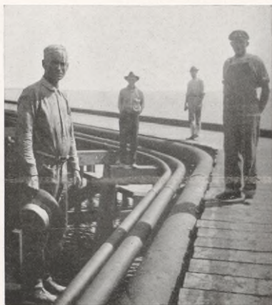
Pipe Line Bend at Dock of Pensacola Terminal
