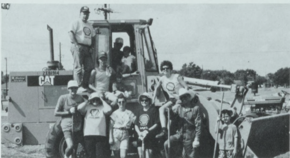
TRACK—With the new jogging/walking track finished, the exercise program at San Jacinto Elementary School in Deer Park is complete. SERVE (Shell Employee & Retiree Volunteerism Effort) along with Student Council and PTO representatives built the quarter-mile track with equipment and manpower furnished by Shell Deer Park. Formed of crushed granite strips, the track circles the school's play park. It will be part of physical education curriculum.
