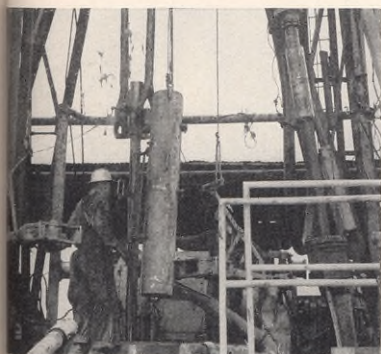
DRILL STEM test, calculated to judge oil producing zone, employs special tool attached to the drill pipe
