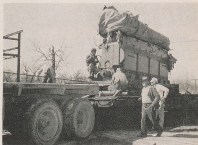
An 800-horsepower engine, weighing 39 tons, is moved from a flat car to a truck.
