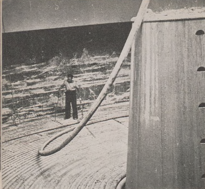
The 3-inch cable carried in the hold of this Liberty ship is in one continuous length for the cross-Channel pipeline.
