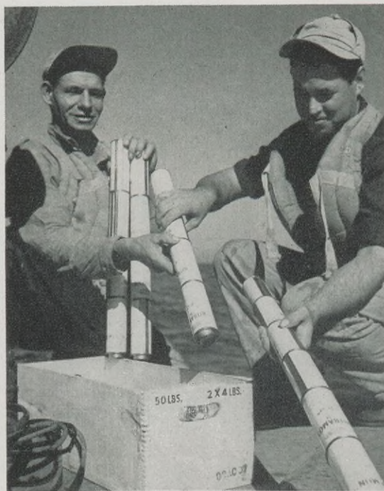
3. From a special barge, a shot hole is drilled in the ocean bottom, and crewmen then prepare the charge to be exploded in the hole by screwing together long, slender cans of dynamite.
