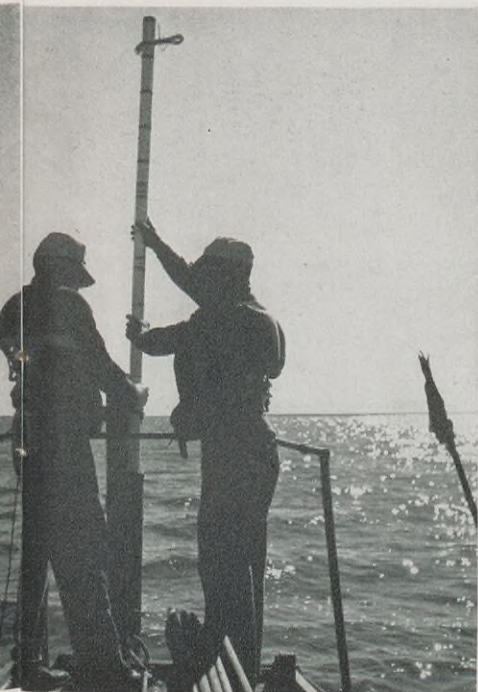
4. The shooting crew lowers the dynamite into the casing which lines the 80-foot-deep shot hole. When they are out of range, the charge will be fired from the shooting boat.
