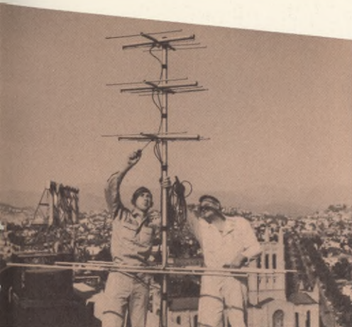
High atop The Town House roof technicians are shown working on the master television antenna which was installed to accommodate all the sets in the hotel.
