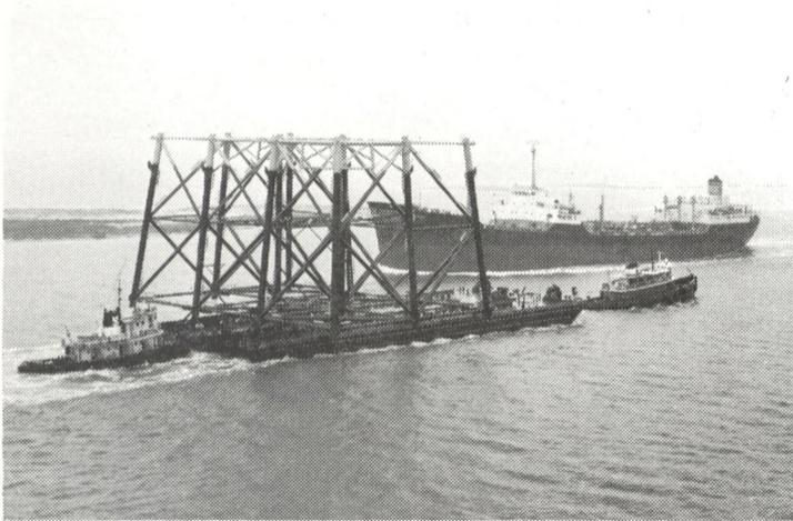
SHELL INSTALLS FIRST PERMANENT PLATFORM in federal waters off Texas Coast. The latest addition in the offshore search for gas and oil are two permanent-type drilling platforms. The trip by barge up the Houston Ship Channel to its location some 30 miles offshore called for some expert navigating. The first platform will be in operation before the year ends and the second sometime during 1965.
