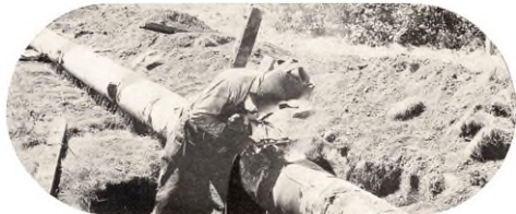
Bellhole Welder on the Texas-Empire Pipe Line
