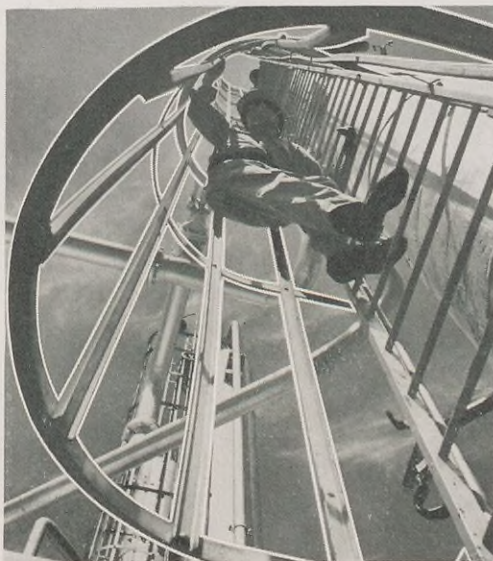
Hazard: Falling. Prevention: A steel "cage" or "basket" surrounds the ladder on a refinery tower to help prevent falls should the ladder climbers lose their footing.
