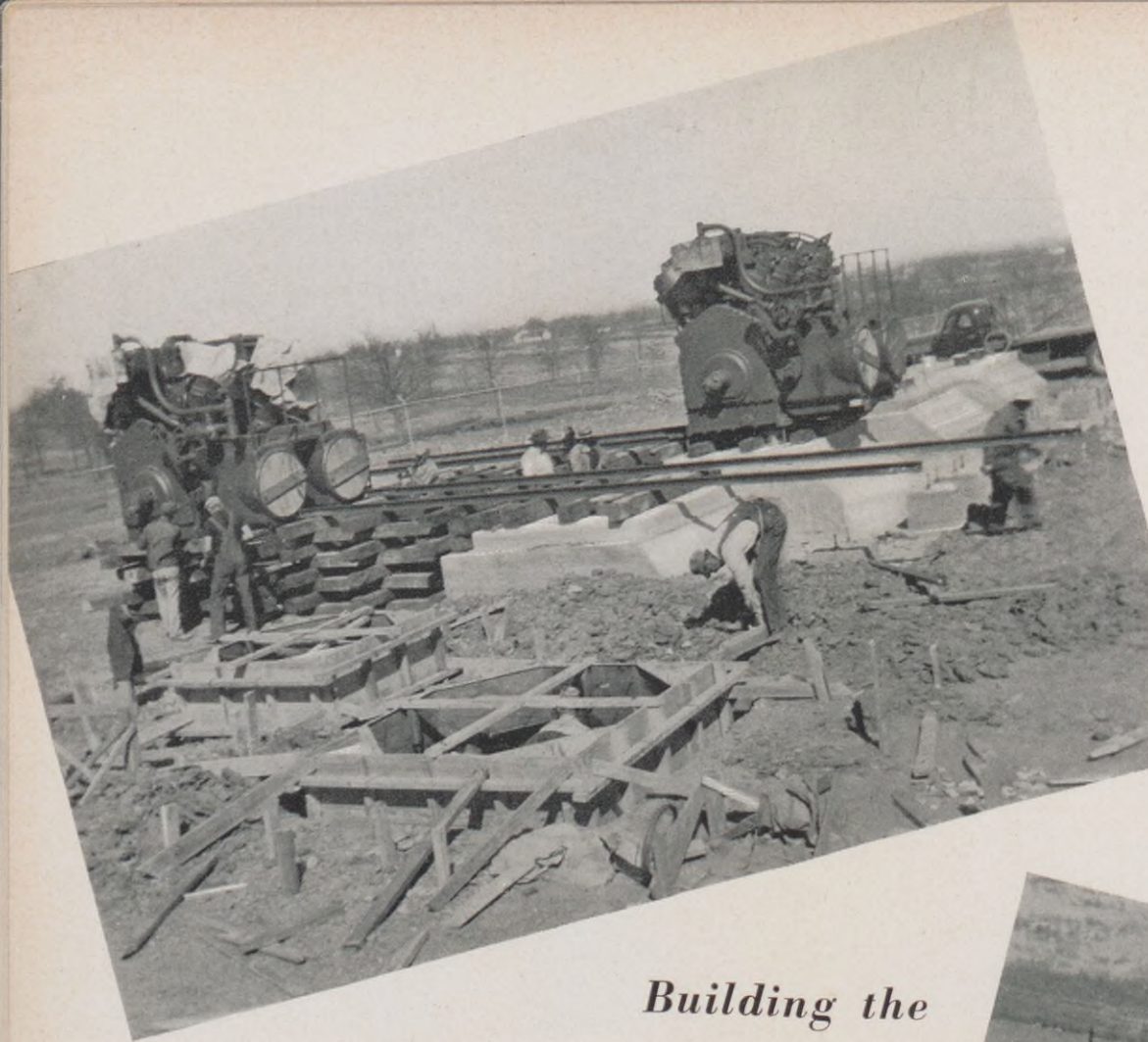
Two of the large compressors are skidded onto foundations.
