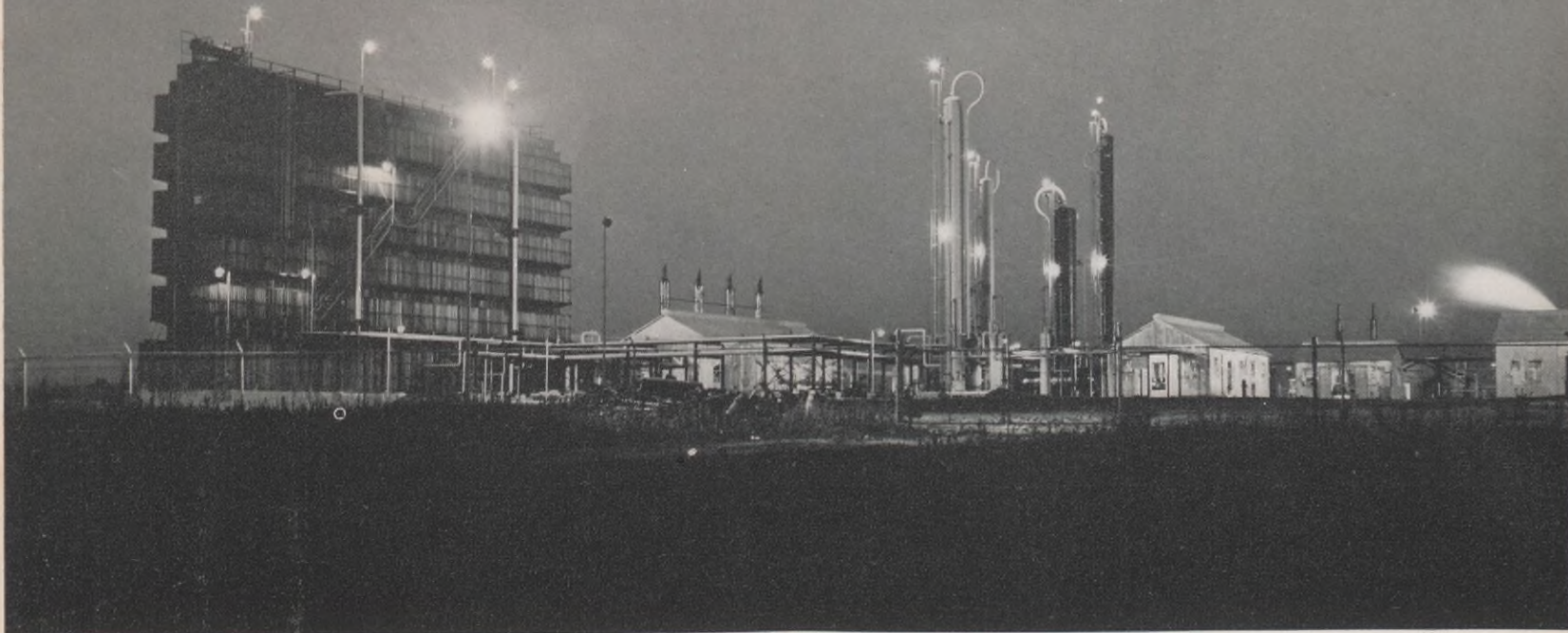
Shell's new East Cromwell Gasoline Plant, the first such plant completed since the war began, produces vital war products without the waste customary in older plants.
