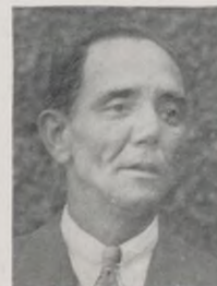
S. P. LIRETTE 20 years November, 1942 Cracking Cleanout Noreco Refinery
