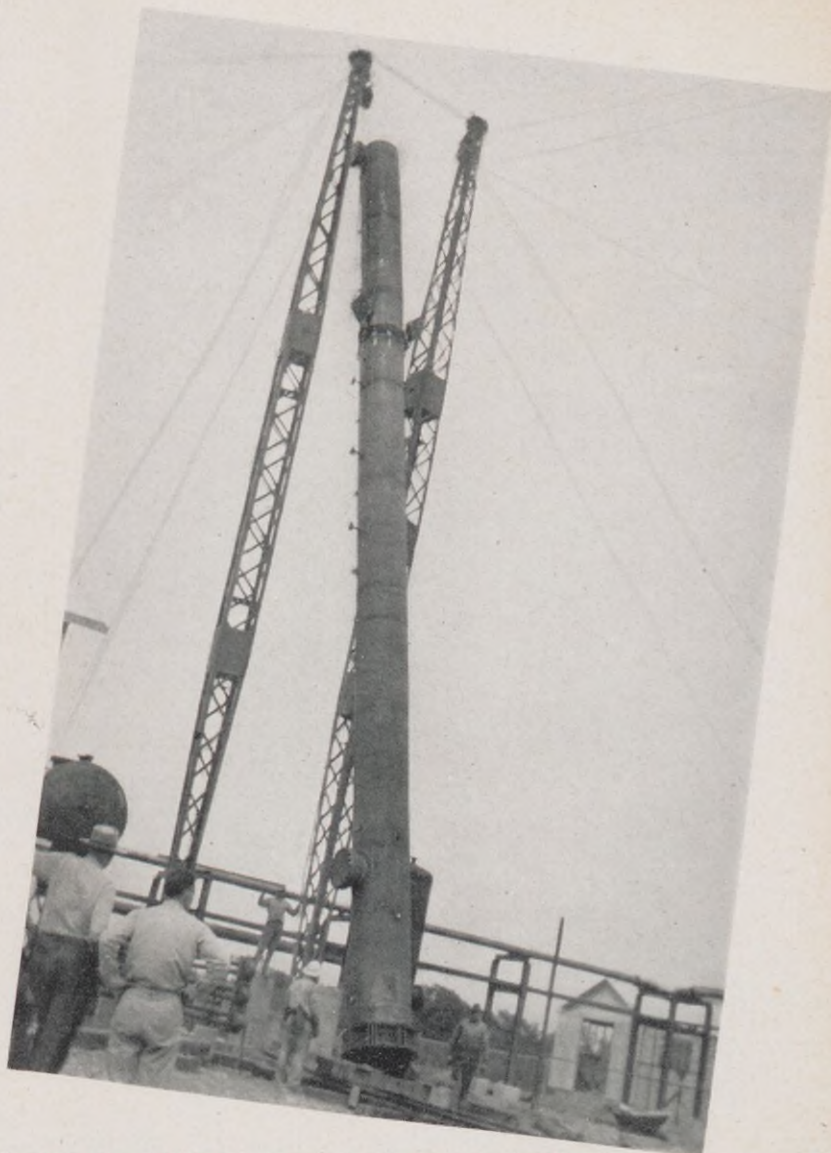
Erecting the stabilizer column at the East Cromwell plant. Mounted on a sled, the column was slid and lifted into position.
