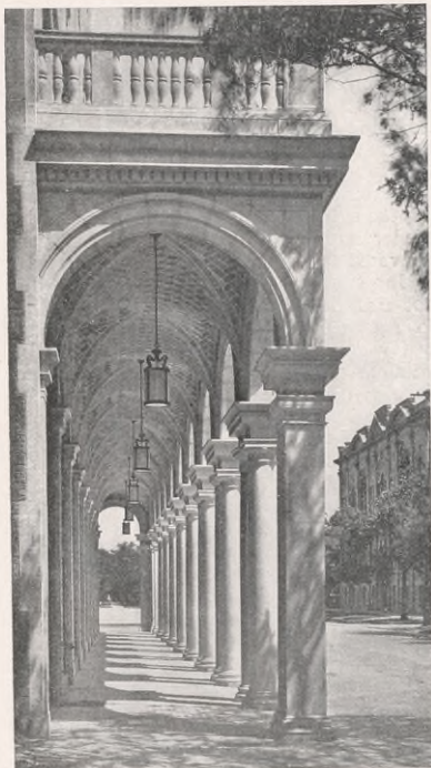
Arcade on Rusk Avenue side of The Texas Company Building, Houston, Texas
