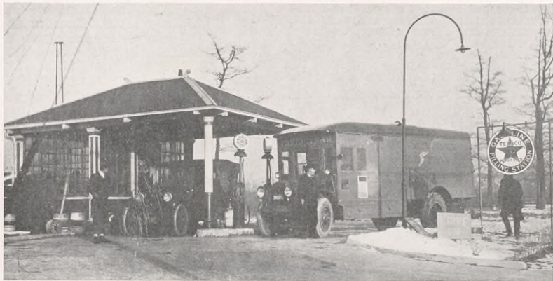
Communipaw Avenue Filling Station, Jersey City, N. J.
