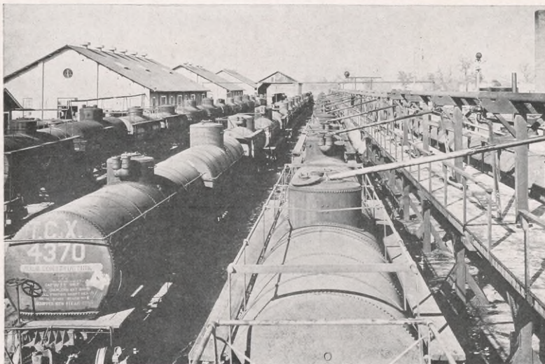
Loading Racks at West Tulsa Works — View from near south end of racks
