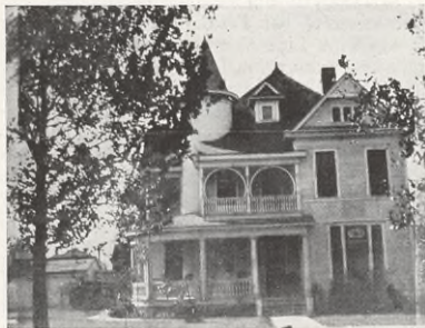
The Texas Club, Calder Avenue, Beaumont, 1902-'05
