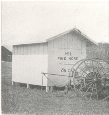
Fire Hose House No. 1, Ludington Lumber Company Green lights burn all night on these houses; they are thus easy to see and hose is always available
