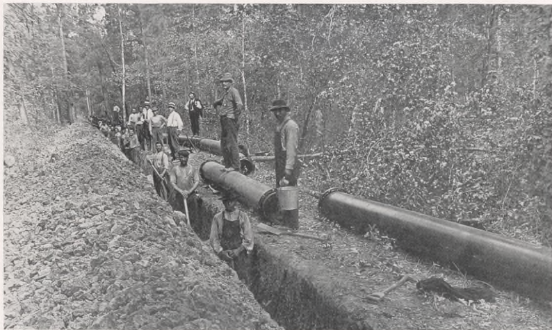
Ditching through woods for gas pipe line
