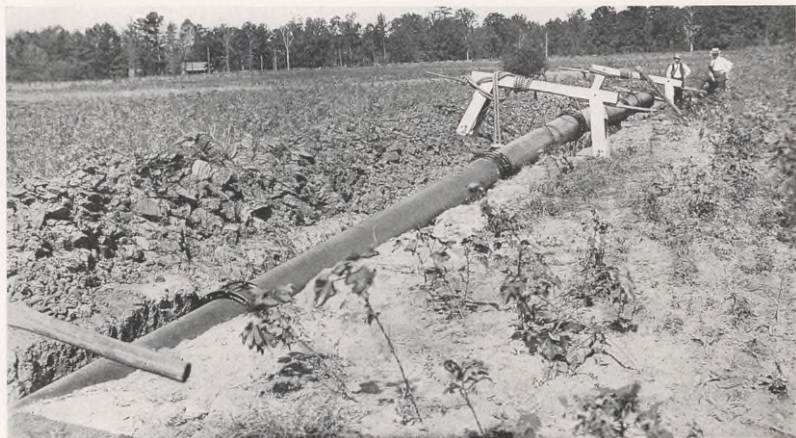
Lowering line into ditch
