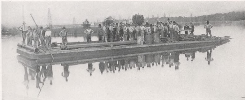
Constructing gas line across lake
