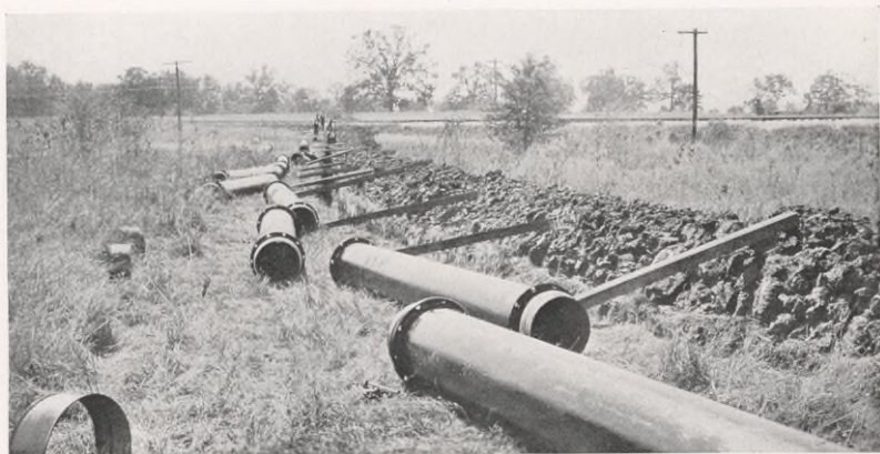
Pipe strung, with couplers in place, ready to be laid
