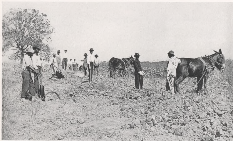
Filling in ditch on 16-inch line
