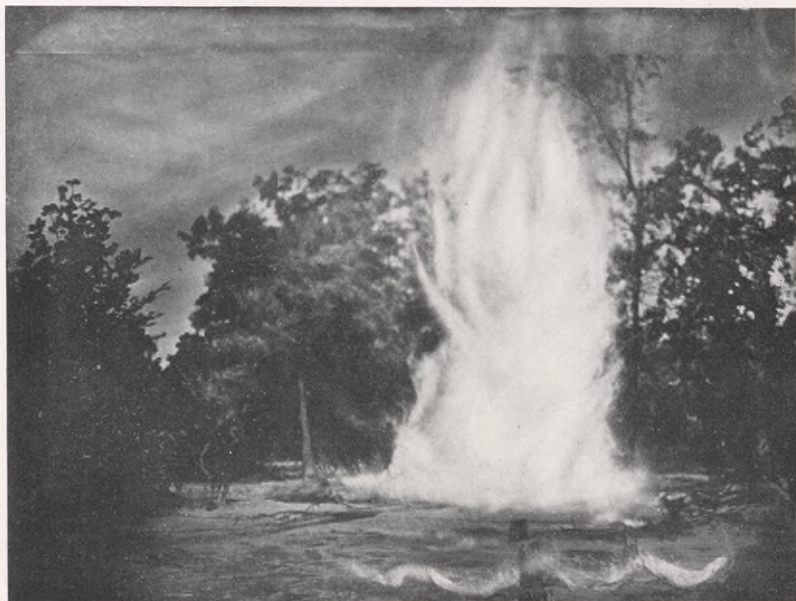
Burning Gas Well. Drilled west of Oil City, Caddo Parish, La., in 1908. Gas blew out around casing, caught fire, and burned continuously for five years until September 29, 1913, when the well was killed by drilling an off-set well and flooding the sand with water.
