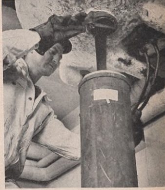
Once mixed, Jato fuel is put into mold to harden
