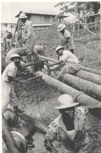
Near Pointe-à-Pierre, above, a gathering line feeding the refinery is re-routed to bypass a new housing development. Below, workers at a drilling site unconsciously display a nimbleness characteristic of the Island's people.
