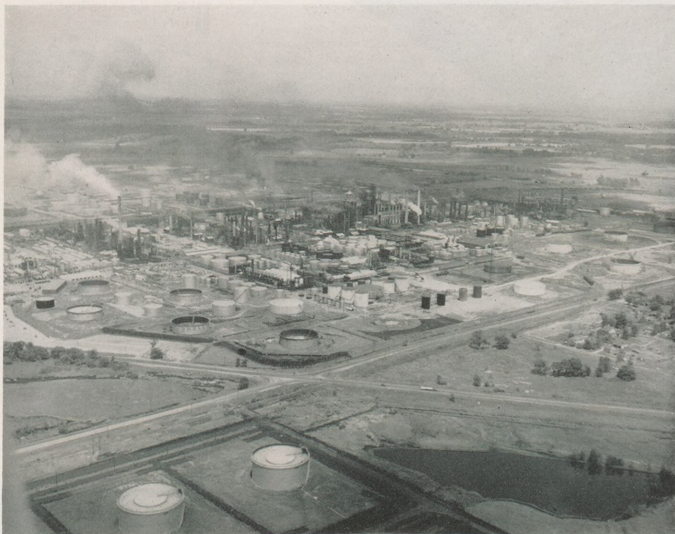
Another 1950 development saw Shell begin work on the design of a new crude distillation plant and other refining units at Wood River. The Refinery's expanded throughput capacity will help Shell meet future increases in demand.
