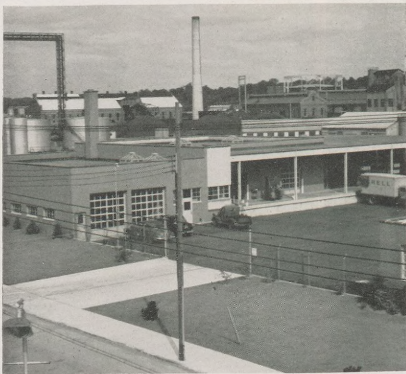
Expansion at Mt. Vernon Depot above was among the major Marketing construction projects completed in 1950. Several long term expansion and modernization projects continued across the country.
