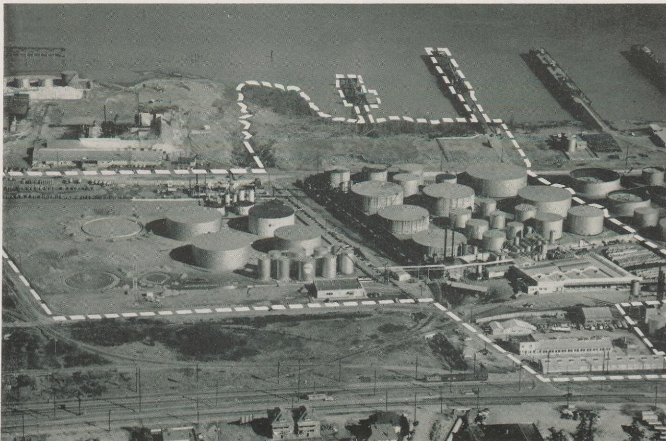
Expanded facilities at the Willbridge, Oregon, Terminal were part of a broad 1950 construction program.
