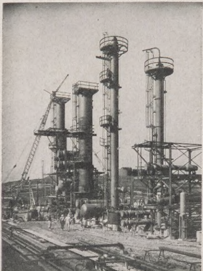
UP goes column No. 2. It's the absorber.
