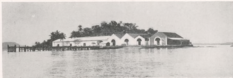
Rio de Janeiro—Ilha Secca Warehouses and Pier
