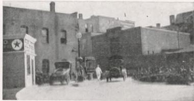
New Street Filling Station, Springfield, Mass.
