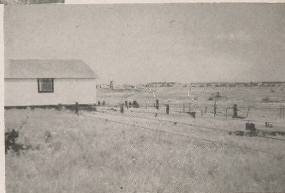
Under the old pumping system now being replaced, a central power plant, right, pulled a series of pull rods to and fro. The motion worked the pumps.
