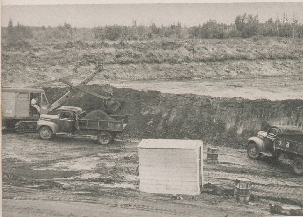
Since the oil sands are near the surface, the easiest method of obtaining them is by strip mining. The scene above is at the Bitumount plant, where the clay, rocks and vegetation atop the sand bed are only eight feet thick. In some areas the layer of oil sand is as much as 200 feet thick.
