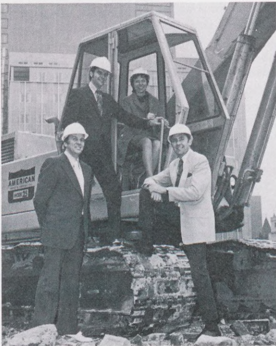
TORONTO PLAZA — Is it a bulldozer in the banquet room or a pile driver in the pantry? Whatever, the piece of equipment pictured is somewhere on the site of the 600-room Toronto Plaza Hotel now under development in Toronto, Ontario. Also on site are hard-hatted hotel staff members, from left- Denis Beaulieu, director of marketing; Jean-Pierre Schweizer, national sales manager; Nan Wrigglesworth, executive secretary; and Michael Lambert, general manager.
