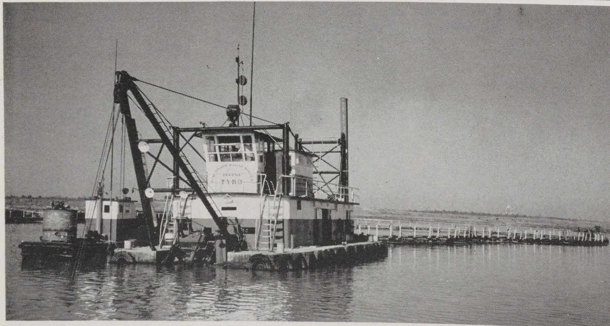
THE KINGFISHER Marine Service's dredge Tyro is seen in action removing silt from the Refinery's docking slip. The snake-like apparatus coming out the rear of the vessel is the discharge line which carries the mud and water mixture to the Jones Lake spoils area.
