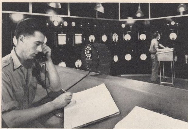
INSIDE THE CONTROL ROOM, dozens of automatic indicators keep the controlmen posted on how the unit is doing
