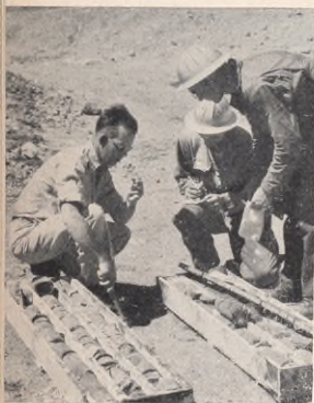
CUTTING SUBSURFACE cores is another method of learning as much as possible about underground formations. Core samples will be sent to a core laboratory to be analyzed for fluid content
