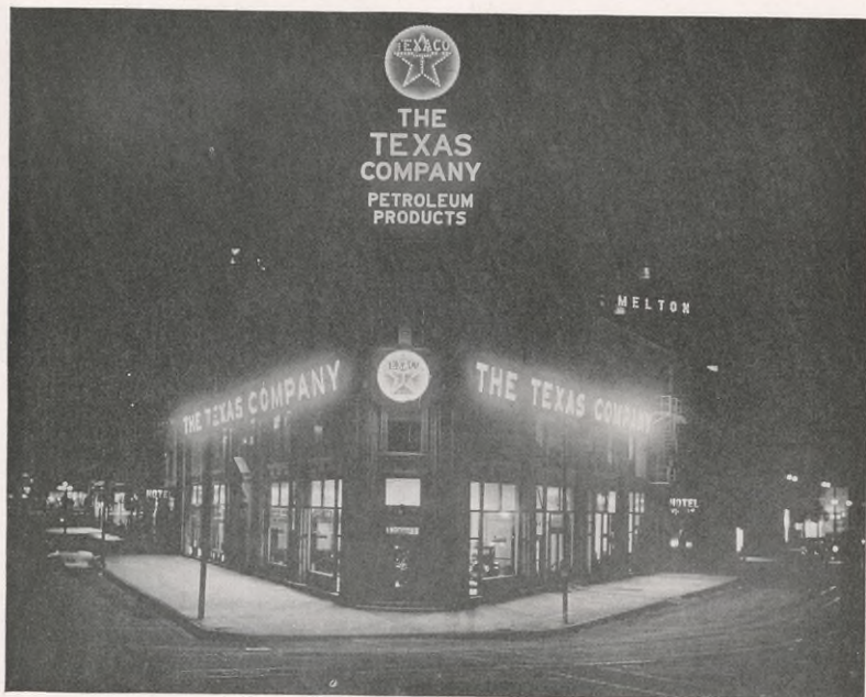
Denver District Office—Photographed at Night
