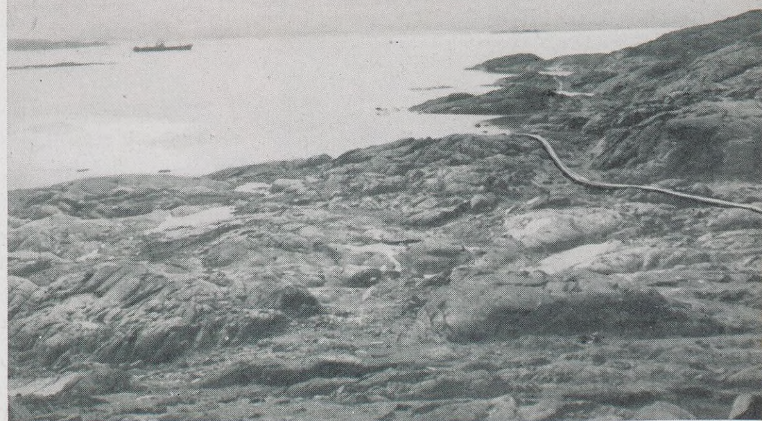
Aviation fuel from Houston Refinery is pumped from ship in the bay through a rubber pipe, seen snaking over rocks at the right, to the Shell of Canada tank, shown below, under construction.
