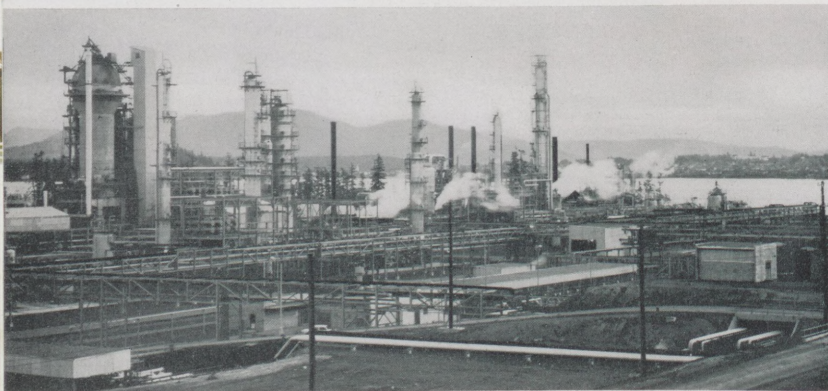
The Anacortes Refinery catcracker unit, far left, which can process about one million gallons of oil a day, was shut down for 30 days last fall for its first overhaul since it went into operation in December, 1955. A catcracker turnaround, which normally is made about every 18 months, gives the opportunity to inspect, repair and improve the unit's operation as a major part of the refinery.
