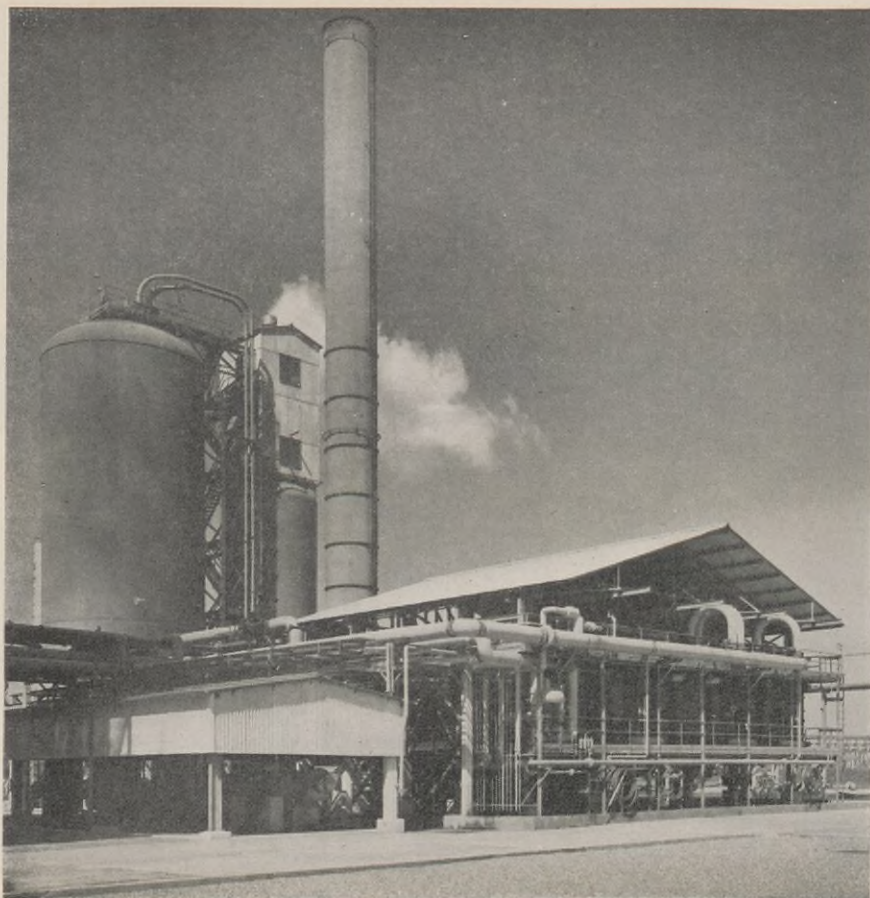
(Left) The heating unit at Houston. Furnace in foreground heats the stock being charged to the cat-cracker.
