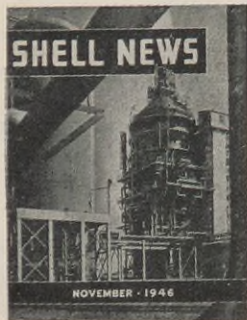
THIS MONTH'S COVER: The catalyst regenerator of the new cat cracker. To the left is the catalyst storage bin. Shaft to the right houses a 15-story elevator.
