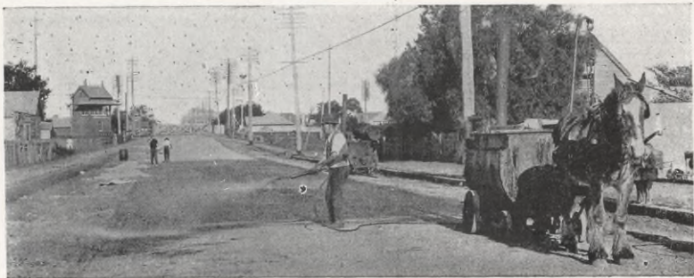
Completing the wearing surface with Texaco Asphalt This road was completed and opened to traffic in May, 1921.
