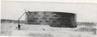
Steel Tank-55,000 bbls. With protection levee, 95% completed, Berwick, La.
