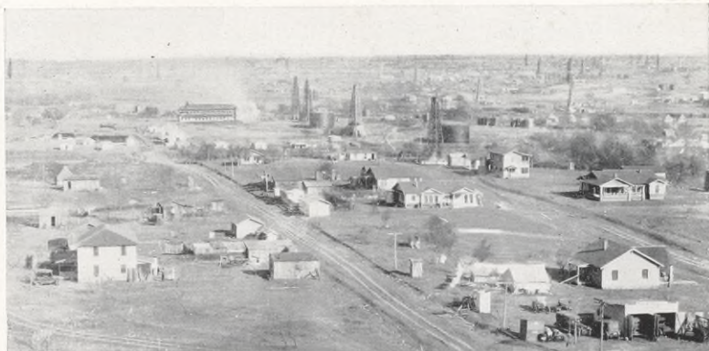
North Breckenridge—From airplane looking east The Texas Pipe Line Company's Pump Station in middle distance at left.
