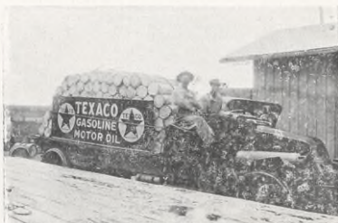
One Hundred Rolls of Tiger Roofing
