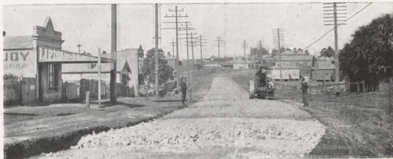
Paramatta Road, showing foundation courses of 11-mile stretch
