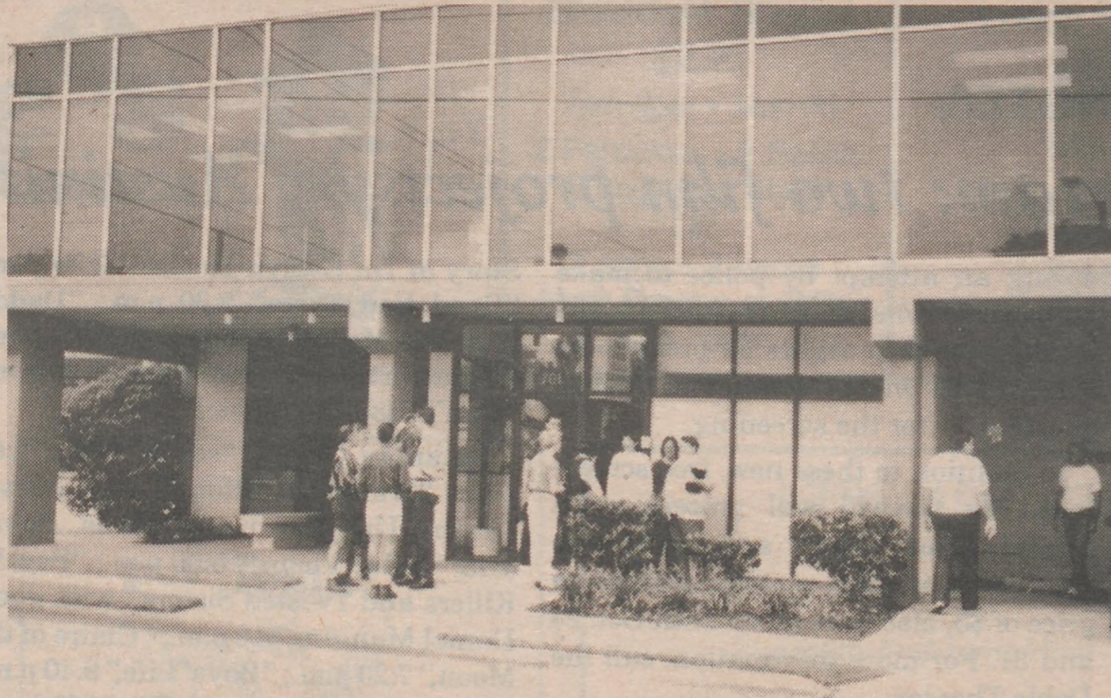
The Montrose Counseling Center's new home at 701 Richmond. The center is scheduled to move on Jan. 22
