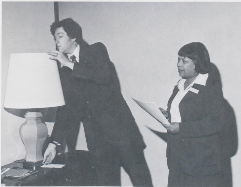
"Maintaining the Product" guest room inspection team at work at the Olympic. At left, Robert Hitchcock, duty manager/trainee, checks out a room lamp light as Director of Housekeeping Shirley Campbell makes a notation on her room item inspection listing.
